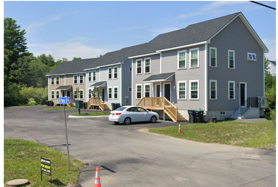
New development of 4-unit multifamily structures at 79 York Street (Google Street View)
