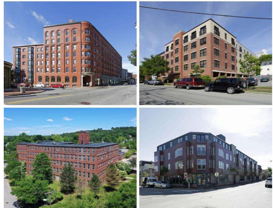
Examples of multifamily housing in Greater Portland
