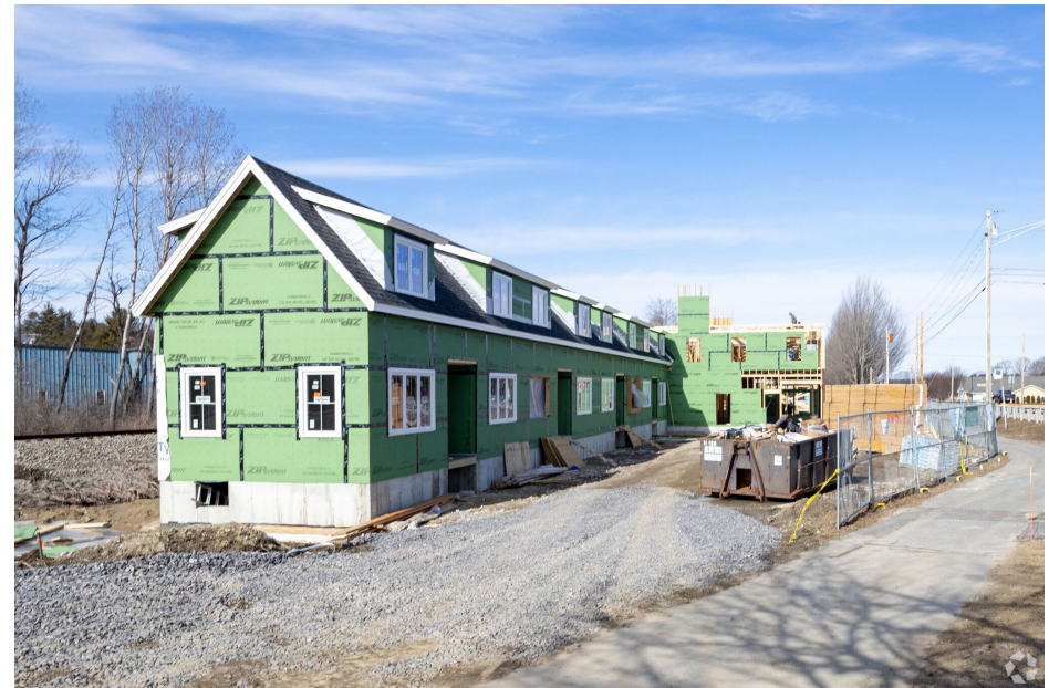
350 Route 1 - Yarmouth Commons, Yarmouth, 18 homes under construction
