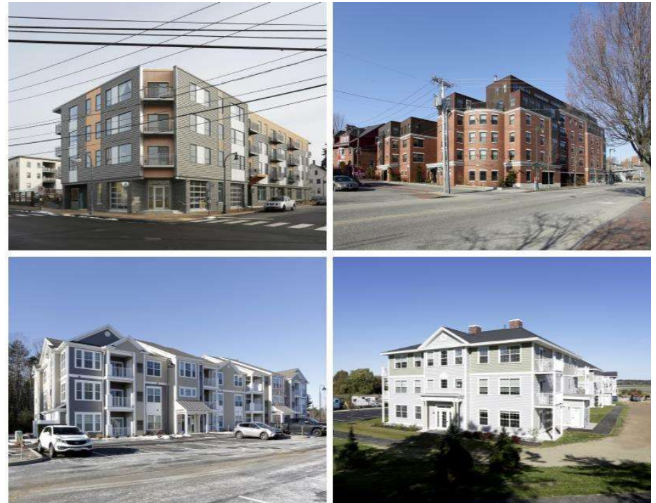
Examples of multifamily housing in Greater Portland
