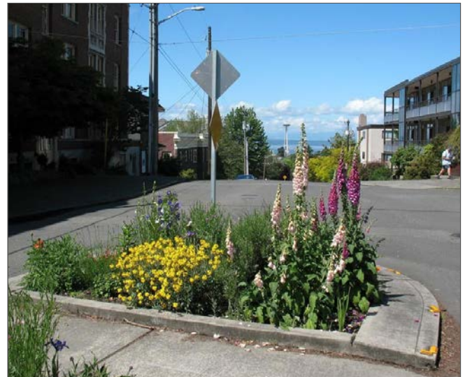
Parking or traffic islands shall be curbed to protect both the pedestrians and the landscaping.
