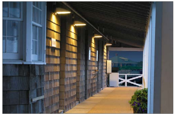
Fully shielded and downward-pointing building lighting conserves energy, minimizes glare, and reduces light trespass and skyglow. Photo by the International Darksky Association
