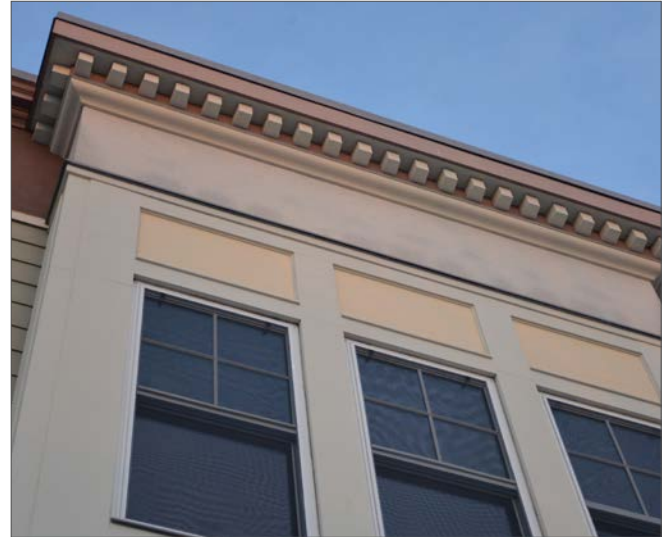
Roof tops shall incorporate distinct features such as roof forms, cornices, eaves and parapets. Photo by Craig Saddlemire
