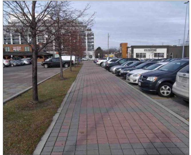
Large parking lots should consider including pedestrian walkways that safely separate pedestrians from vehicles. Photo by Bob Topping/DesignABLE Environments
