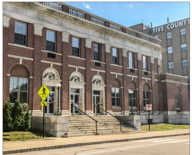
Additions at either end of the Post Office duplicated the arched window bays and continue the belt course.
