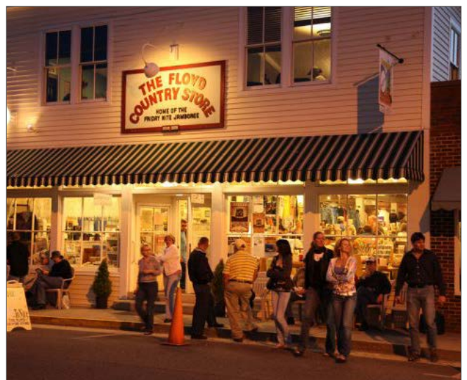
Building façades may be illuminated with soft lighting of low intensity
