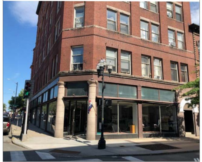
Lisbon Street's ground floor shops have recessed entrances, clerestory windows, intermediate cornices, and large windows.
