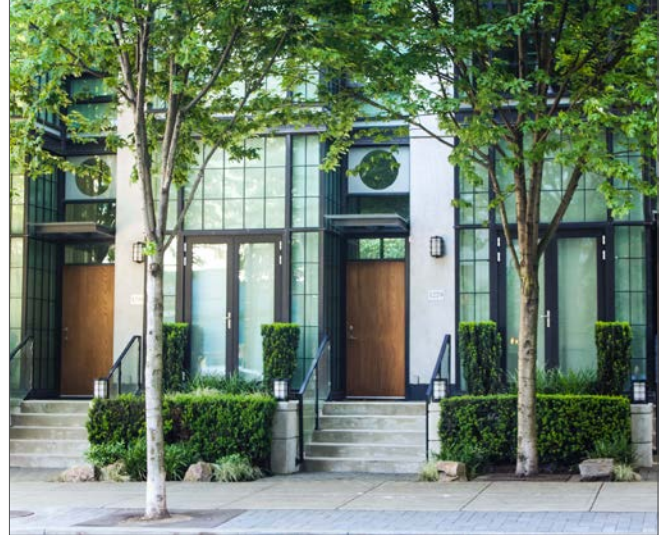
Ground story dwelling units shall be elevated at least 21 inches above the grade of any adjacent sidewalk.
