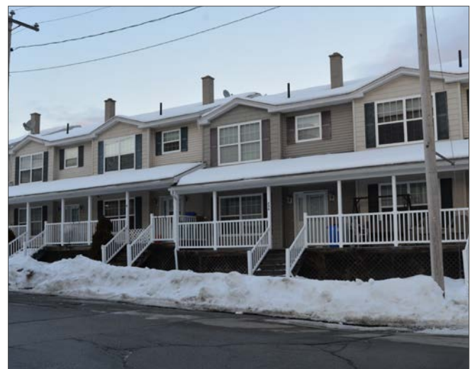
Roofs shall be designed to prevent falling ice and snow onto entrances and walkways. Photo by Craig Saddlemire
